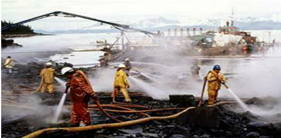
Figure 2.6: High Pressure, Hot Water Washing in Shoreline Clean Up (Source: Exxon Valdez Oil Spill Clean Up Methods, 1993)
